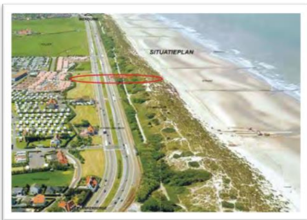
Photo 11 Situation trussgirder bridge Wenduine
