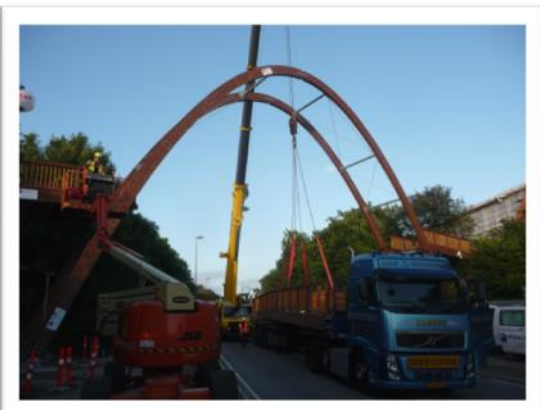
Photo 8 Setting up the bridge sections
