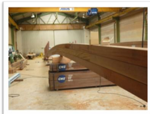
Photo 3 Dowel laminated bridge beams
