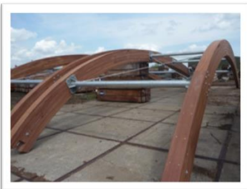
Photo 2 Dowel laminated arches
