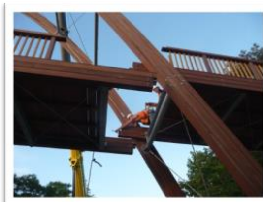
Photo 9 Setting up the bridge sections
