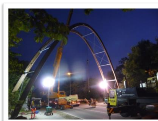
Photo 7 Setting up the arches
