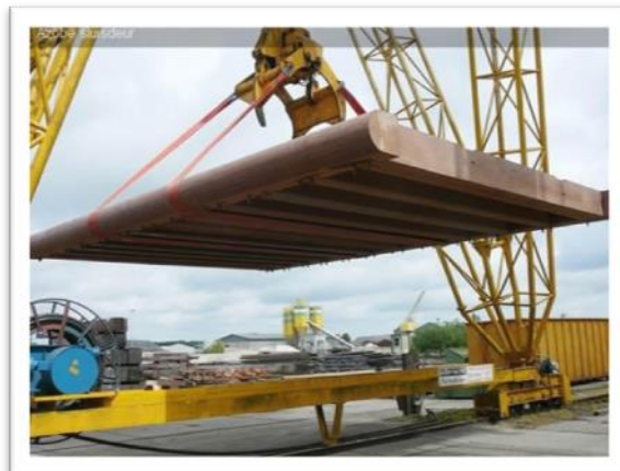
Photo 17 Timber floodgate horizontal
